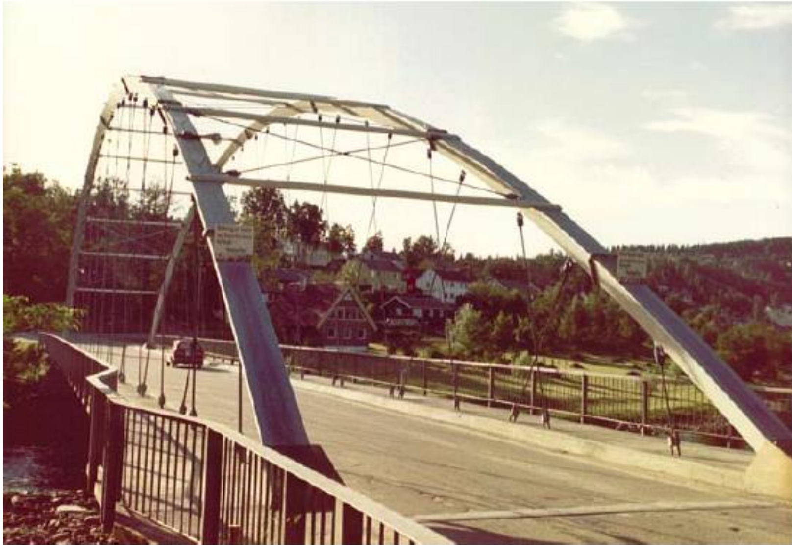
Fig. 7. Bridge at Steinkjer, Norway, built 1963-1964
