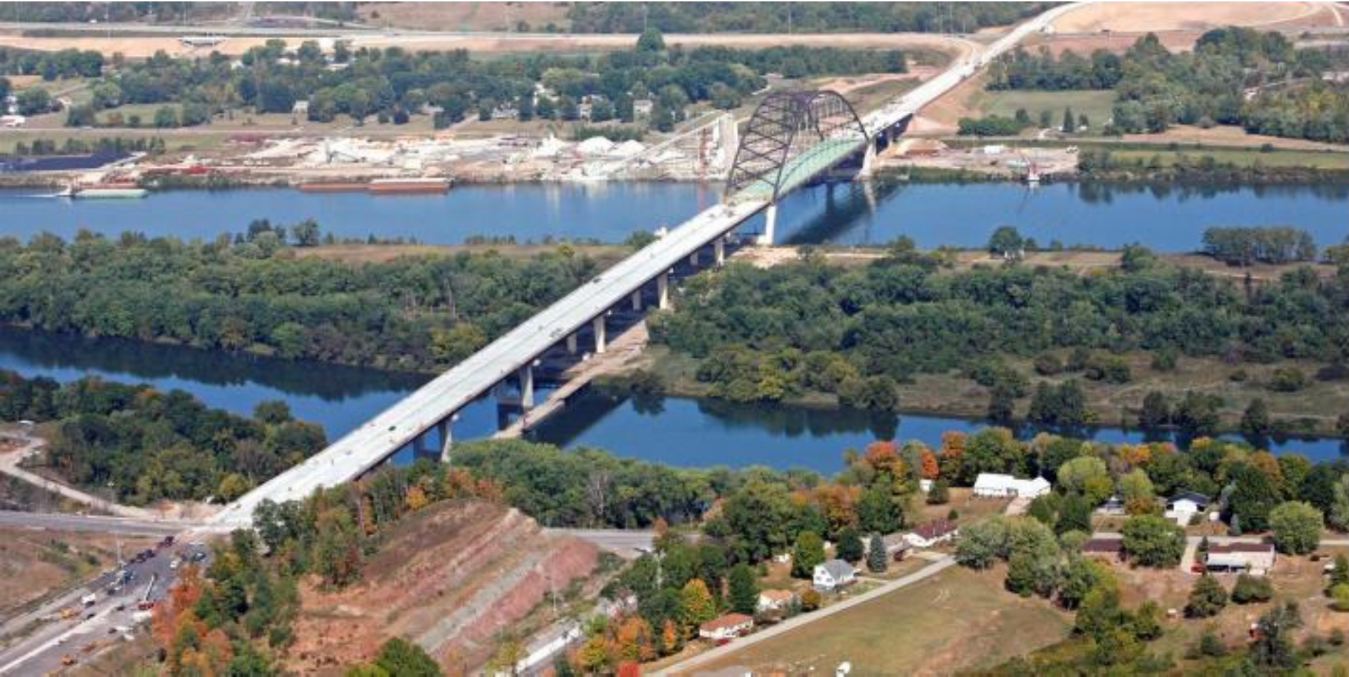
Blennerhassett Island Bridge , 268m
