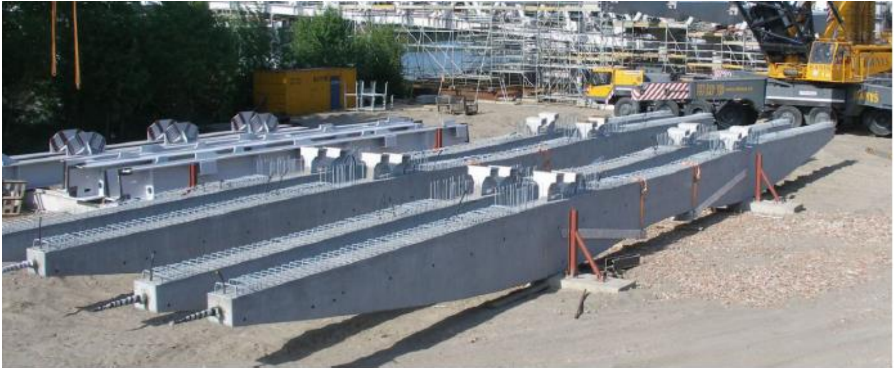
Fig. 4 Precast transversal beams stored on the site prior to assembly
