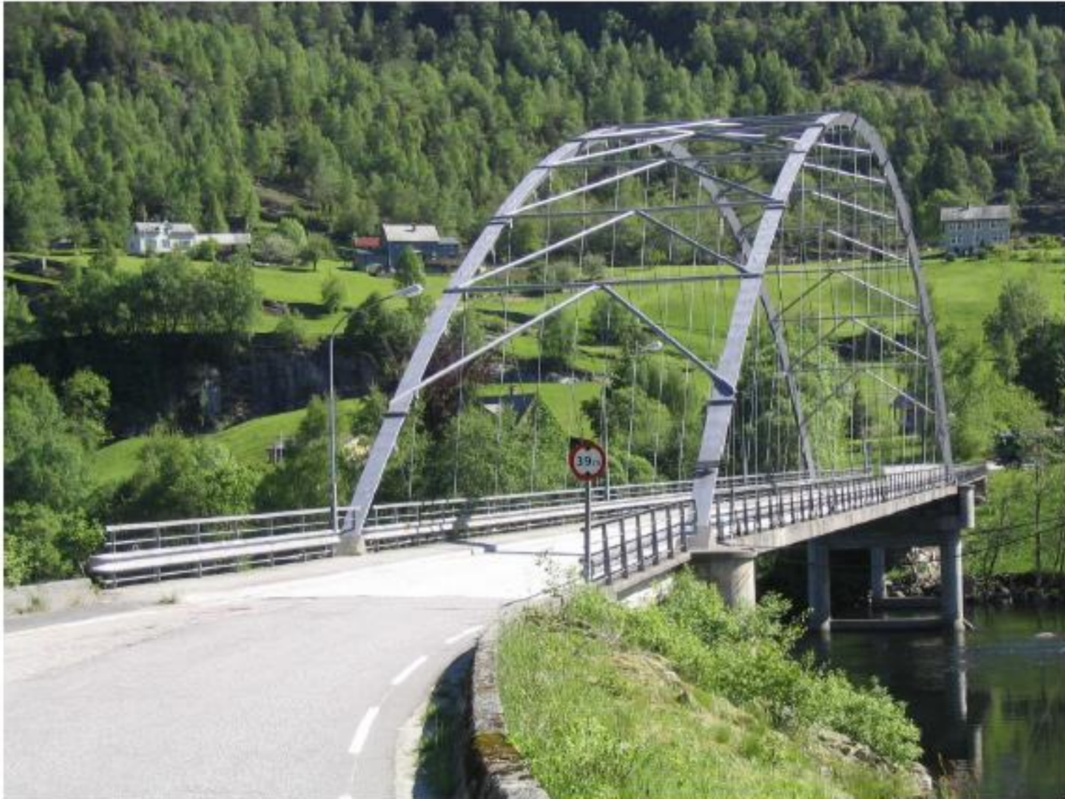
Fig. H5. The Bolstadstraumen Network Arch seen from the south
